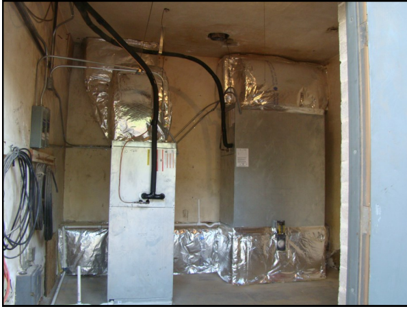
Our NEW Heat Pump systems for the lodge building — a major investment for our lodge building, completed in July
